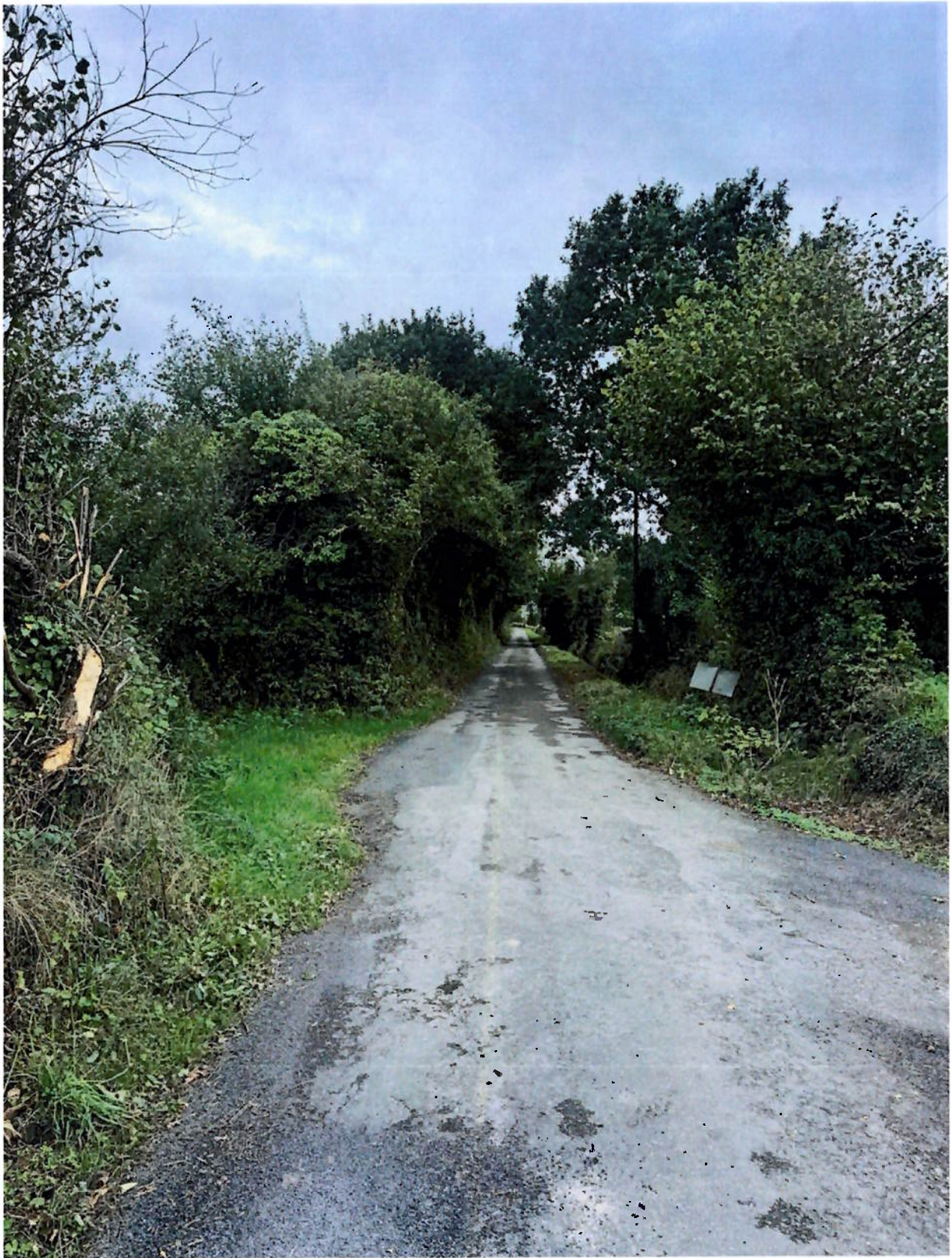
Photograph 3. Representative view showing the very narrow carriageway with mature hedgerows and trees immediately adjoining both sides and little or no usable verge.
