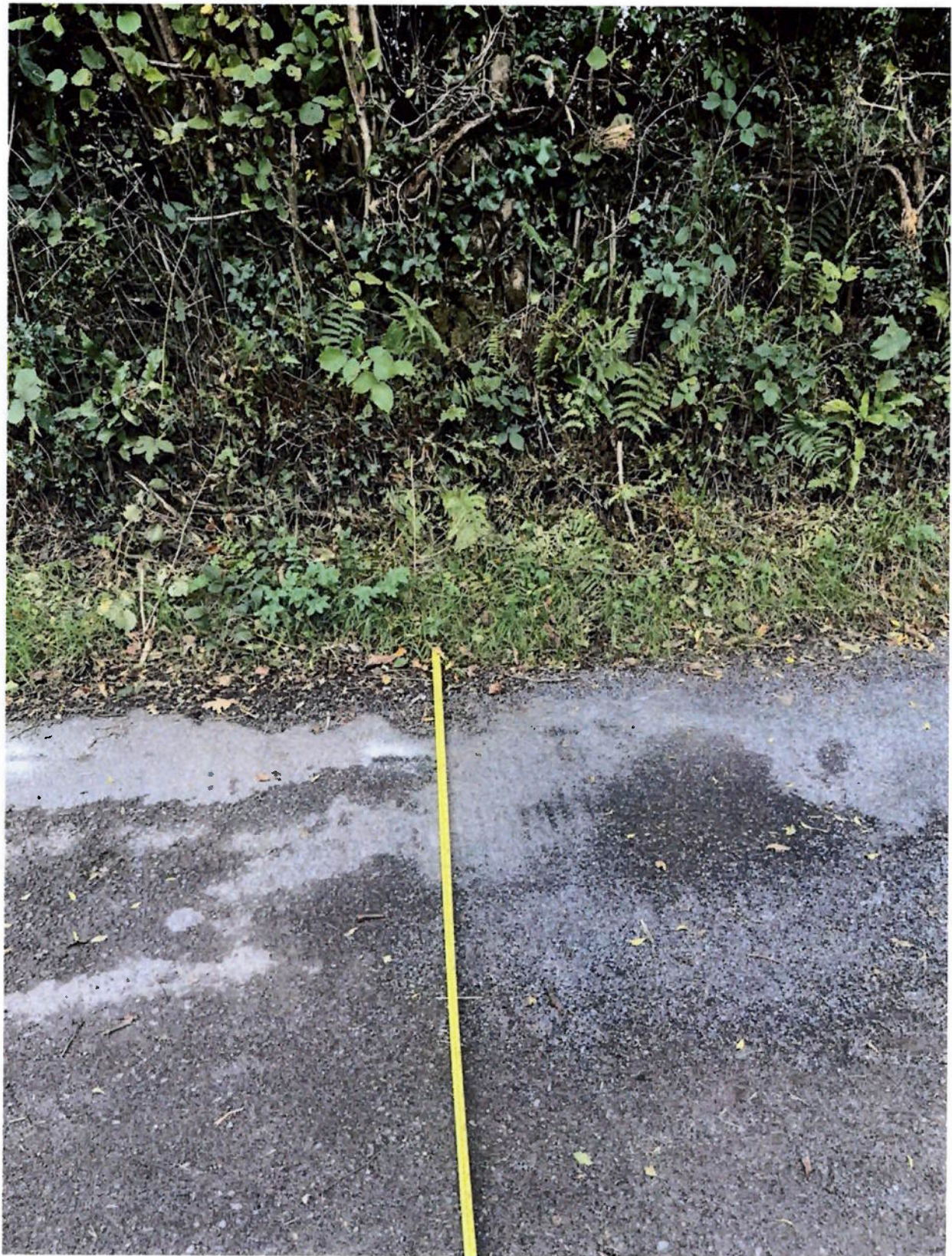
Photograph 2. Road-width measurement at a representative point. The affected road is approximately 3.2-3.3 metres wide at the measured location, and its narrow character is broadly replicated along the approximately 1.3 km cable section.
